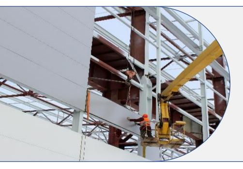
ALC Panel or Autoclaved Lightweight Aerated Concrete panel is composite material consists of cement, lime, and silica sand. These panels use two-way welded steel mesh as reinforcement
